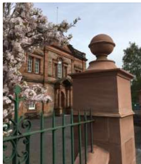
Victoria Hall Gate Piers
