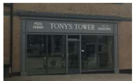
Replacement Traditional Style
