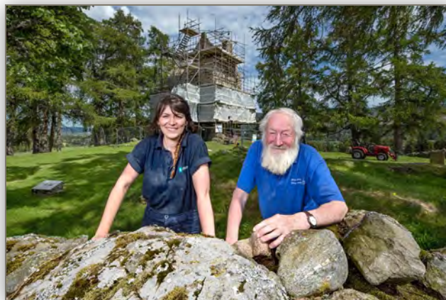
Conservation work at Knock Castle
